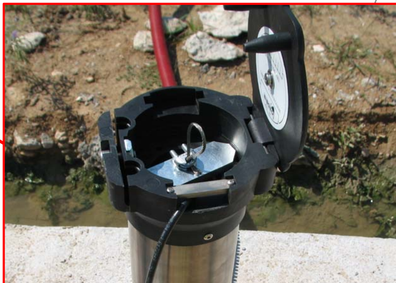
Support top cap after installation
