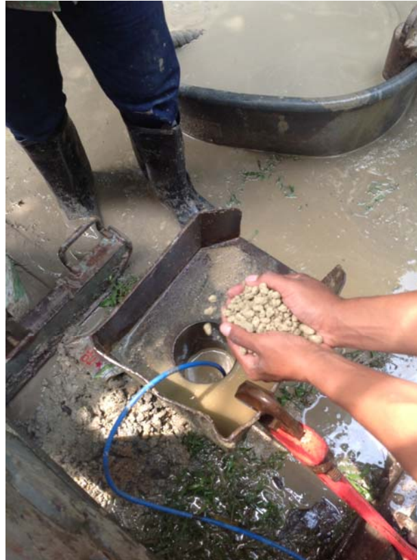
Filling with bentonite pellets (sealing)
