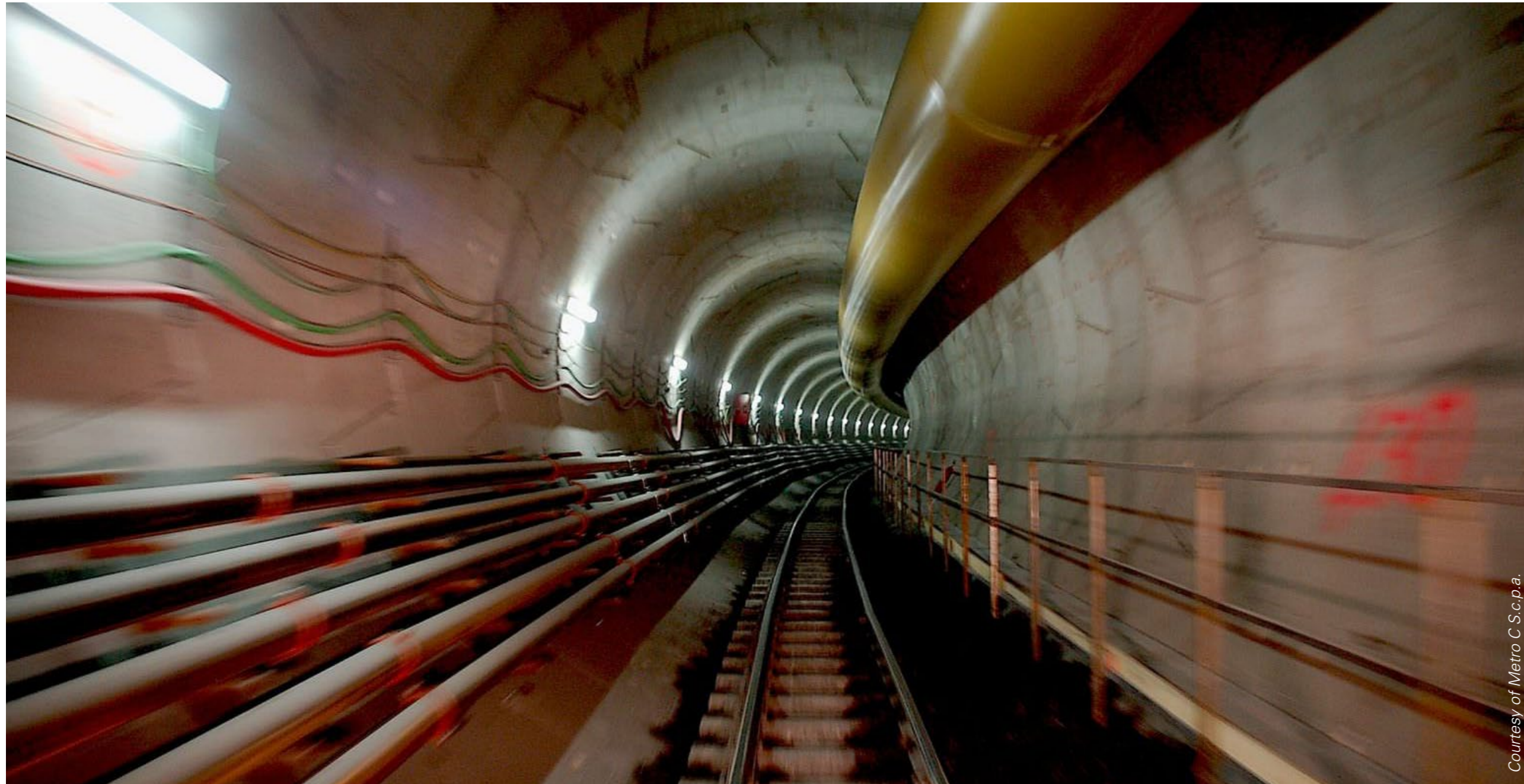
New Line C tunnel excavated with TBM machine. Concrete lining are instrumented with Sisgeo vibrating wire strain gauges
