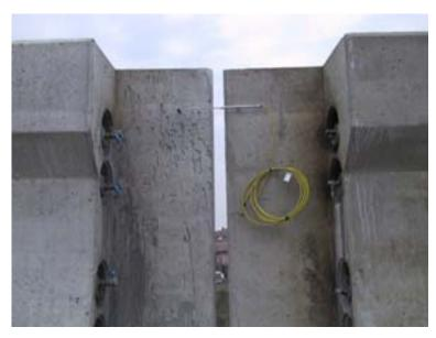
The instrument applied in bridges is used for the control of the movements of joints between decks or to control the movements between support and bridge deck.
